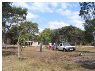
Preparing the site for the container
